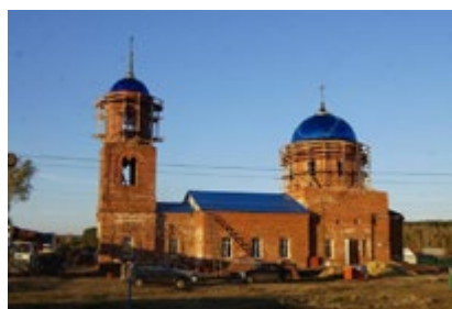
After the restoration
