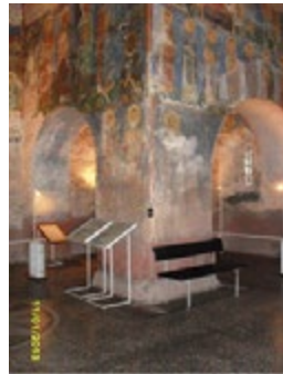
Figure 3 – Heating of the Cathedral with portable electrical heaters.
