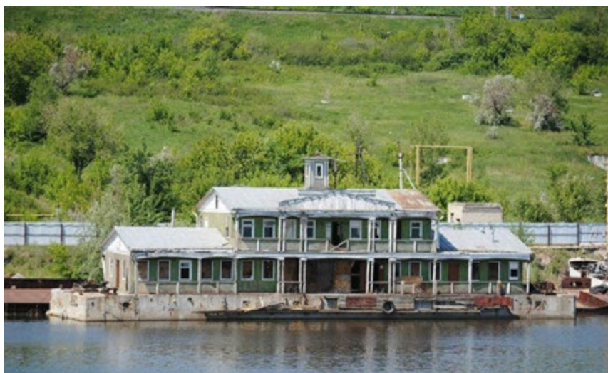
Figure 2 – landing station. Project 47B. Photo of 2015
