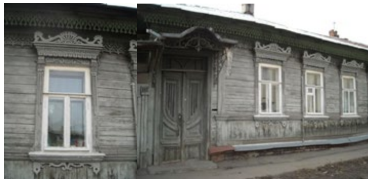
Figure 6 - Dwelling house with a wooden cladding on a stone base in Orel at 2-nd Pushkarskaya, 29
