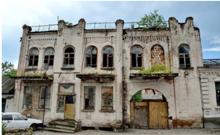
Figure 7 - "the House with chains"
