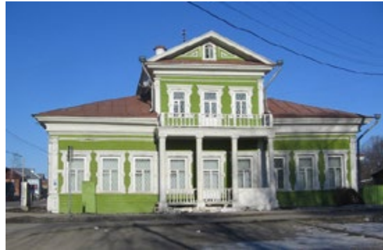
Figure 12 - Wooden house with walls with boards cladding in Yakutsk.
