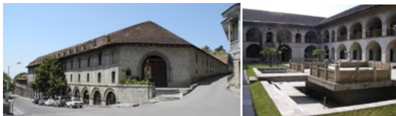
Figure 7 a,b - The upper caravanserai in Sheki
