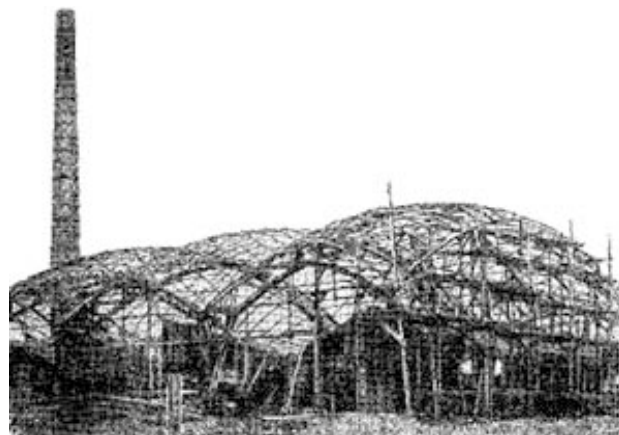
Figure 4 – Spatial covering of double curvature on a rectangular plane in Vyksa (1898)
