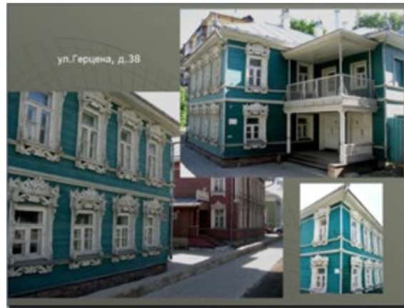
Figure 8 - Wooden log house with planking, built in 1825.
