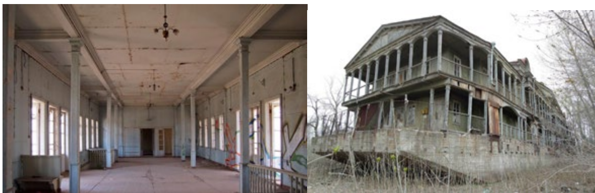
Figure 5 – landing stage for Lake Denezhnoe. Interior of the hall
