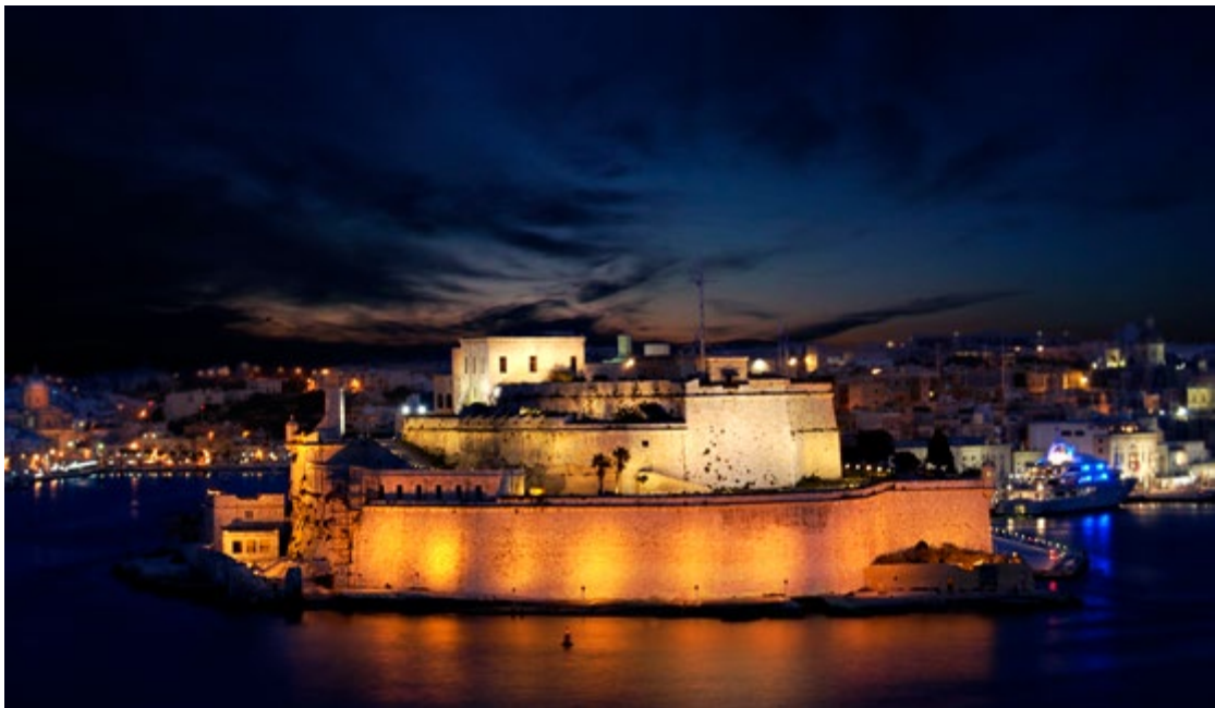
Figure 3 - Fort St.Angelo in Birgu recently restored
