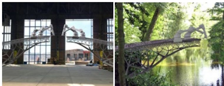
Figure 4 –Amsterdam’s new 3D-printed steel bridge
