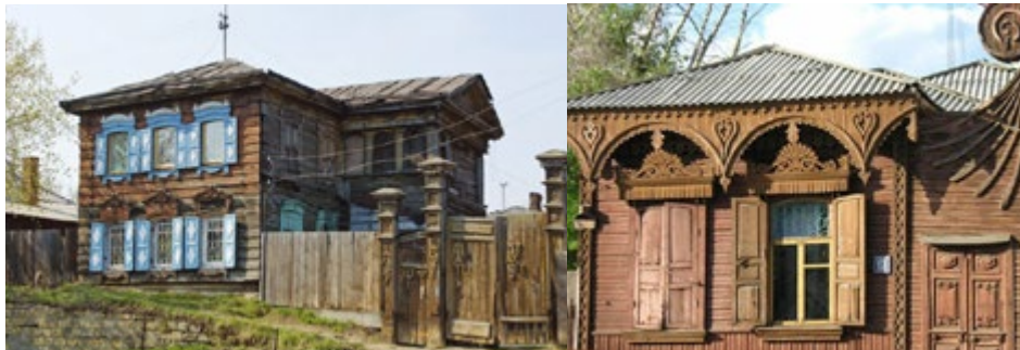
Figure 13 - Wooden houses in Yakutsk. The external walls made of logs with board cladding
