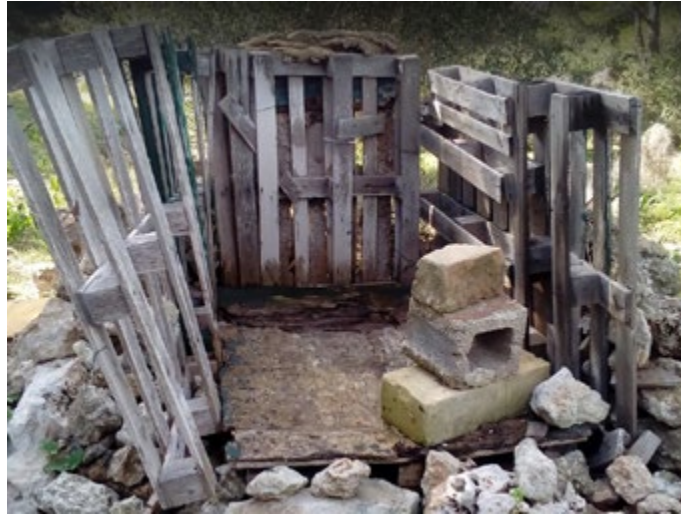
Figure 2 -Vandalised gun hide in St.Paul`s Bay
