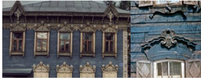
Figure 11 - Wooden house in Irkutsk. The external walls made of logs with board cladding and the facade is decorated with carvings.
